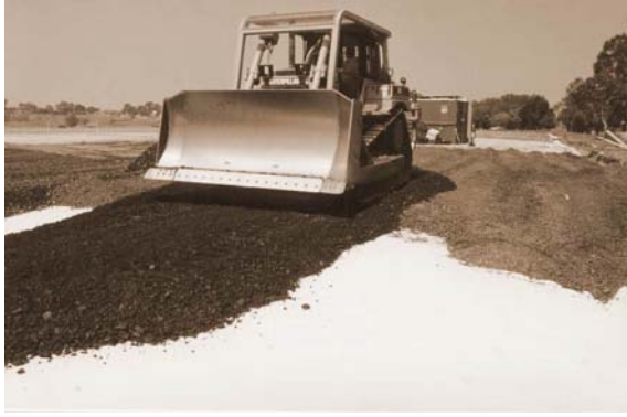
Figure 5: Placement of 300 mm cover layer over the GCL cap.
