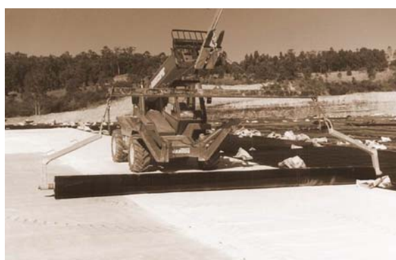
Figure 1. GCL installation completed followed by HDPE.
