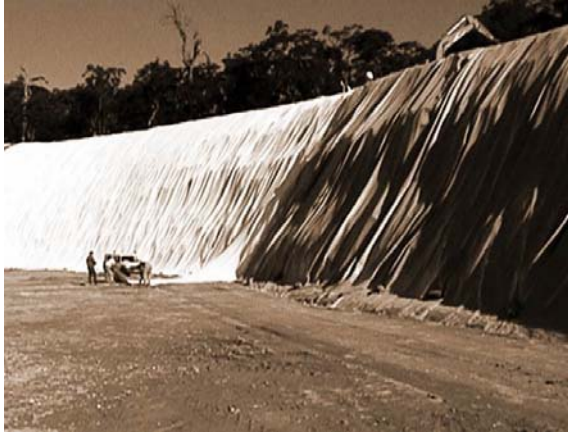
Figure 8: Cushioning fabric installed followed by GCL.
