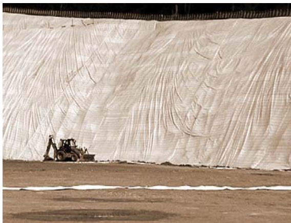
Figure 7: Steep wall lined with cushioning fabric, GCL and semi-permeable membrane.
